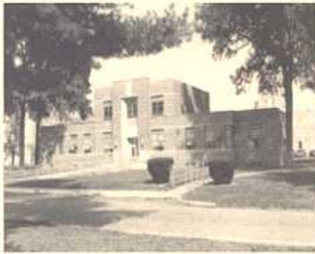
Administration Building, Muscatatuck. Photo by Glenn Mather, October 2004.
