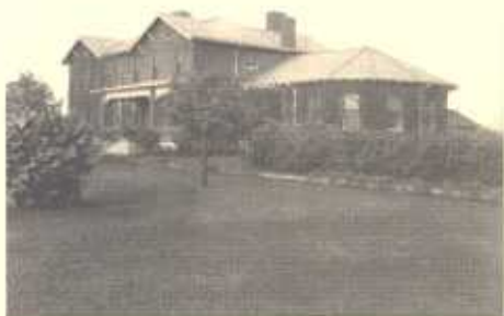
White Building in Colony II at New Castle
